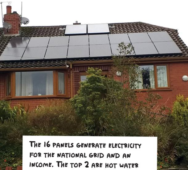
**THE 16 PANELS GENERATE ELECTRICITY FOR THE NATIONAL GRID AND AN INCOME. THE TOP 2 ARE HOT WATER SOLAR PANELS. - PHILIP**
